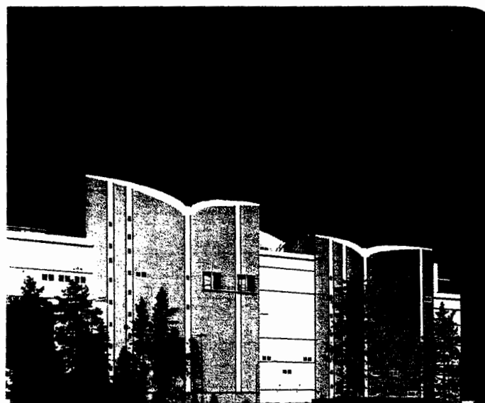
Dáva district heating and power station Umeå, Sweden entered service in 2000. The fuel source includes municipal refuse. Photo: Von Roll Inova
