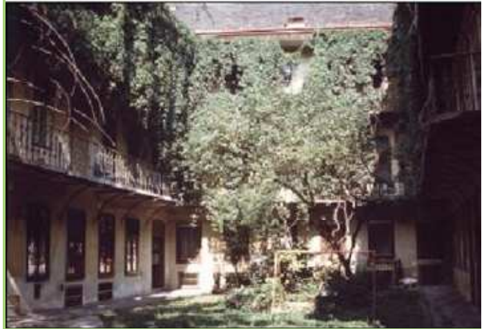
Cortile a giardino in condomino
